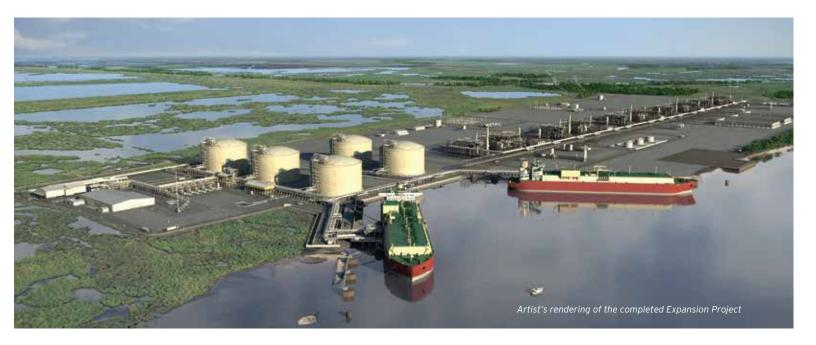
Cameron LNG's Expansion Project is capable of increasing LNG production capacity by 9.97 million metric tons per annum (Mtpa) of liquefied natural gas (LNG), or 1.41 billion cubic feet per day (Bcfd).
